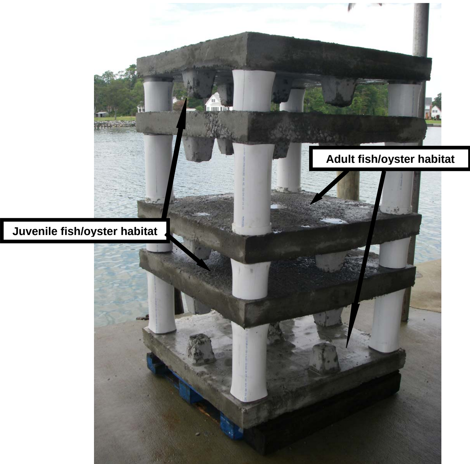
Figure 3. Constructed artificial fish reef. Twelve have been deployed at two VMRC reef sites, Northern Neck and Poquoson.
